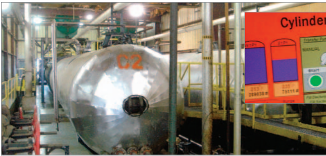
Installation of additional cylinders...
